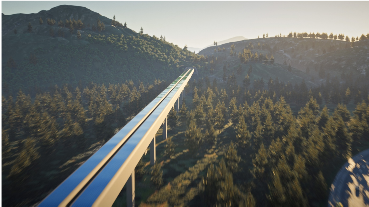
Figure 2: A rendering of a hyperloop system with solar panels covering the top of the tube.
