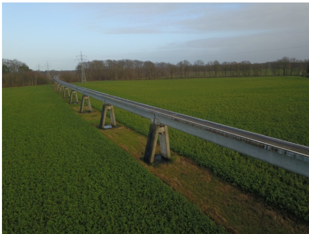
Figure 3: TVE in Lathen with existing support structure and uninterrupted 32km test track
