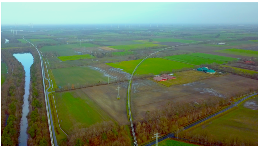
Figure 1: 32km MagLev Transrapid test facility Emsland, Lathen, Germany (TVE)
